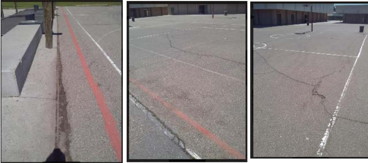
**The recommendation for the blacktop to the east side of the quad area is to have it seal coated and restriped. This will require cutting out some areas (as the first picture indicates) and replacing that asphalt to clean up the edge.**
