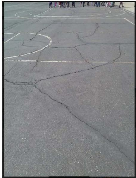
In this 3<sup>rd</sup> picture there are actually little pieces breaking off and the broken pieces are being removed from the cracks by the students, causing trip hazards.
