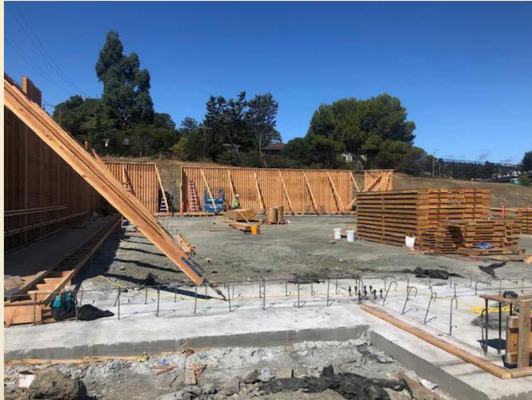
Framing for the shoring of the hill at 36 th and the Abbott Driveway
