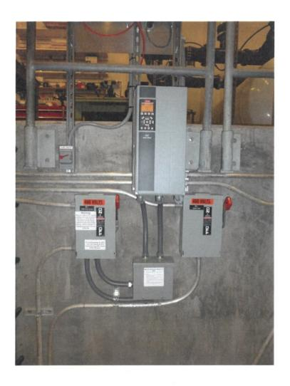
22 KW / 30 HP, 380 - 480 VAC, Three phase, IP55 / Type 12
