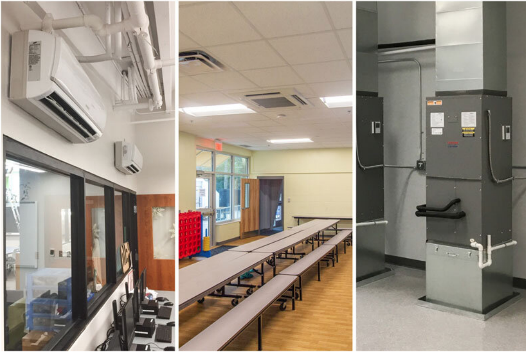
K-12 school classrooms are primarily conditioned by three different types of indoor units: high wall mounts, ceiling cassettes, and ducted air handlers. Pictured VRF equipment by Samsung , Mitsubishi Electric , and Toshiba Carrier .
