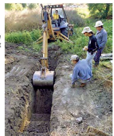
Trenching across the Hayward Fault in Fremont
