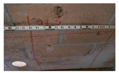
The existing concrete slab-on-grade was also tested to determine if reinforcing steel was present. As depicted by the red lines in the photograph to the right, the slab-ongrade has reinforcing placed in two directions. However, the reinforcing steel size and placement within the slab thickness could not be determined.
